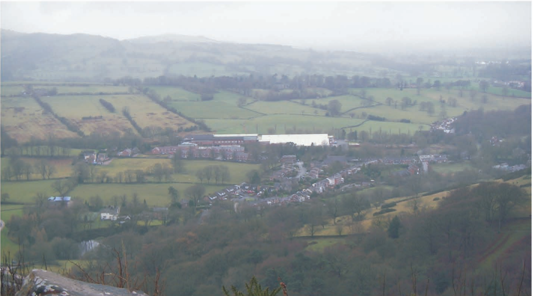
Existing view showing the visually intrusive roofs of the Langley Works
